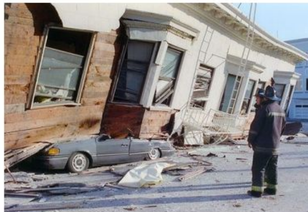
Photograph of destroyed buildings after earthquake
