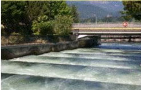
Fish Ladder at the Bonneville Dam on the Columbia River Separating Washington and Oregon
