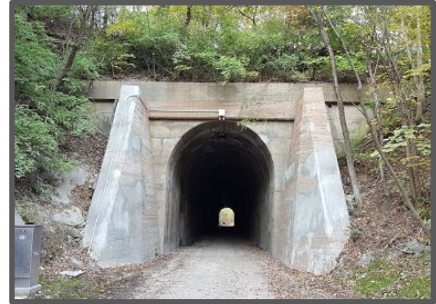
Vale Tunnel, KCMO
